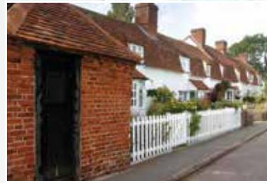
Caidge Cottages and former lock-up
