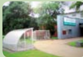
* Under cover cycle park facilities at Beverley Leisure Complex
